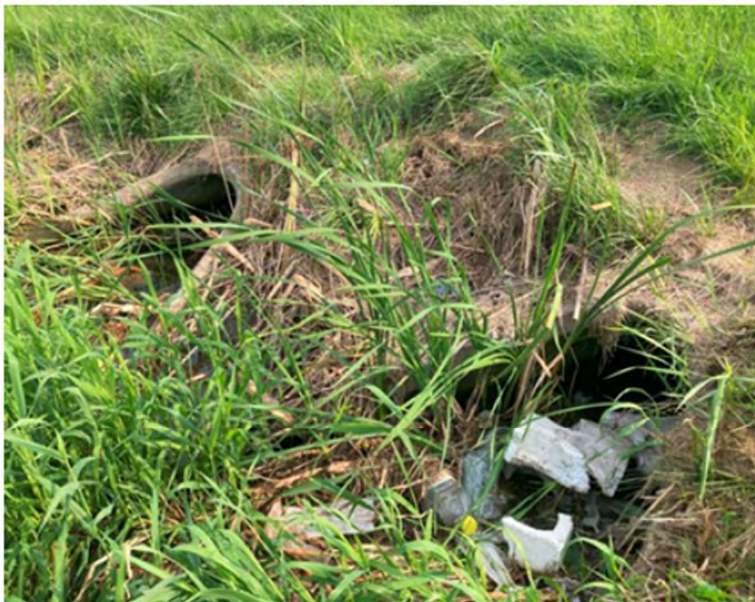
Figure 1. 24" inlet pipes. Minor debris and vegetation were noted during the time of inspection.
