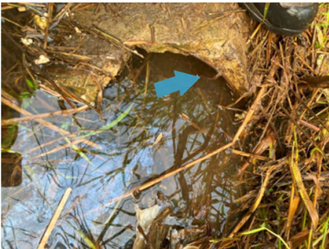
Figure 2. 12" principal spillway inlet with an ~8" section of missing concrete causing exposed reinforcement as depicted near the arrow.
